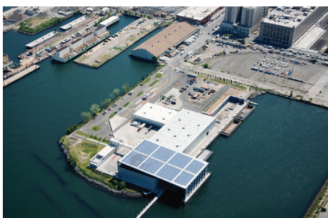
The Sunset Park Materials Recovery Facility is located on the Sunset Park waterfront in Brooklyn.
